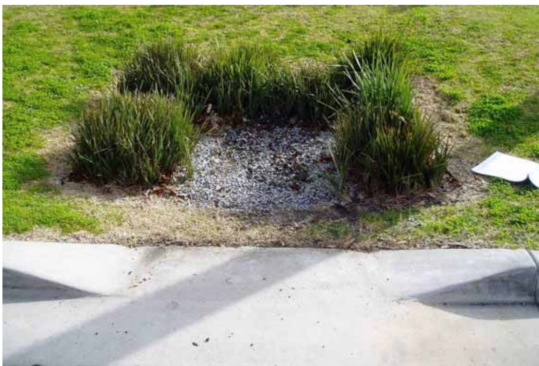
Figure 3-12 A single layer system that includes an area where the planter bed has been inserted, Riviera Street, Mentone
