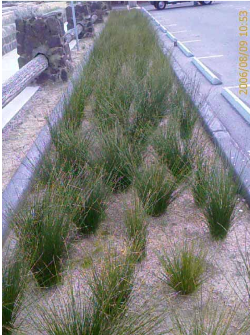
Figure 3-7 Rain garden with concrete edge beam, Ricketts Point, Beaumaris
