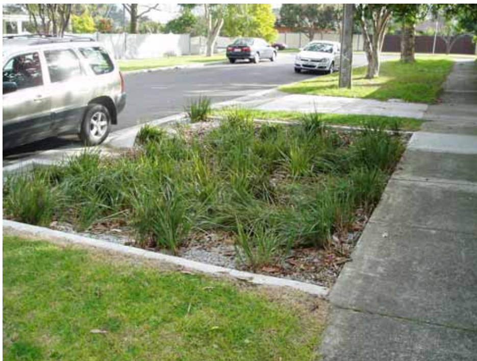
Figure 3-10 Concrete edge strip used to delineate a rain garden, Stawell Street, Mentone
