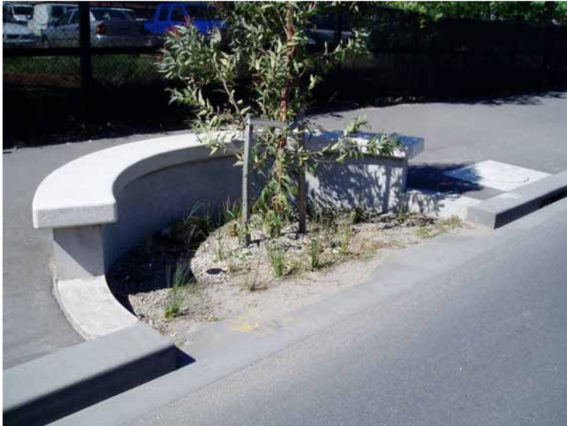
Figure 3-9 Seating used to accommodate the grade change at a rain garden, Docklands
