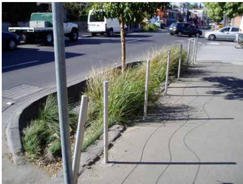
Figure 3-2 Damage to fences, Cremorne Street, Richmond
