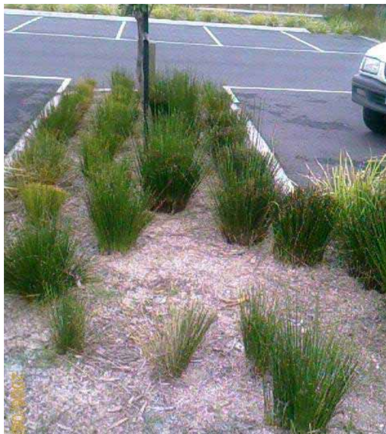
Figure 3-22 An example of plants that have been trimmed excessively
