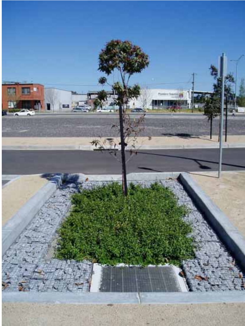
Figure 3-8 Edge details at Point Park car park, Docklands
