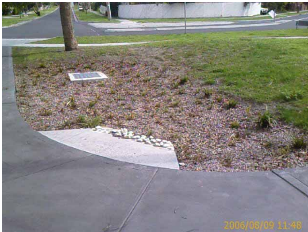
Figure 3-5 Mulched and planted batters, Voltri Street, Cheltenham
