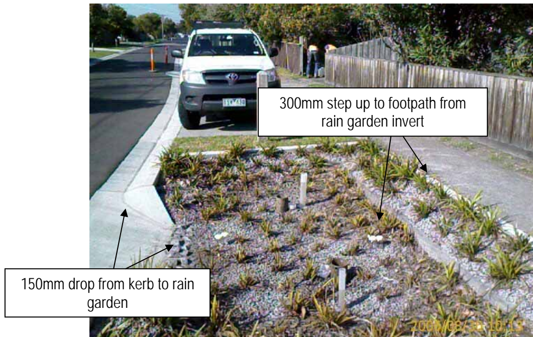
Figure 3-3 An example of the grade change to be accommodated across a rain garden, Alleyne Avenue, Chelsea
